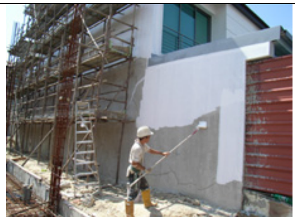
QUICSEAL 103 ECO for external wall waterproofing
