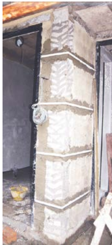
1. QUICSEAL 409 set with mortar base
