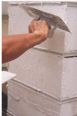
2. Plastering wall to finish flush with plasterwork trim
