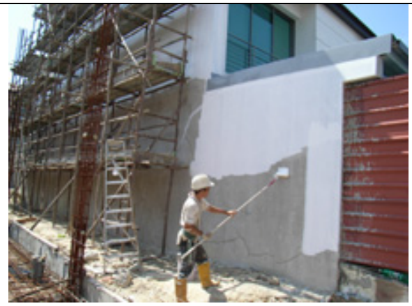
QUICSEAL 103 ECO for external wall waterproofing
